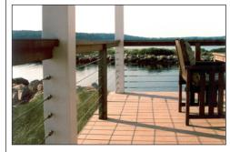
(A) Threaded Terminals connect cable through the post via a nut or end cap.
